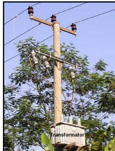
Gambar 5.9 Transformator Distribusi Tipe Tiang
