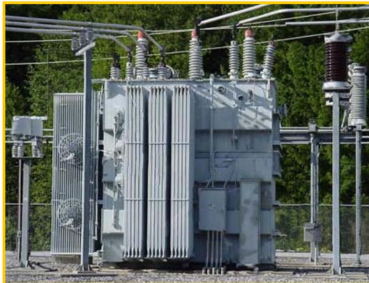
Gambar 5.8 Transformator Daya
