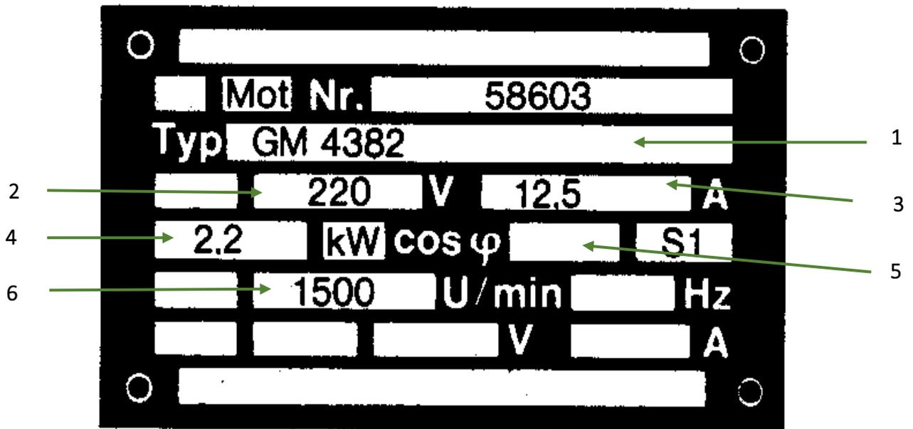
Gambar 43. Nameplate motor DC
