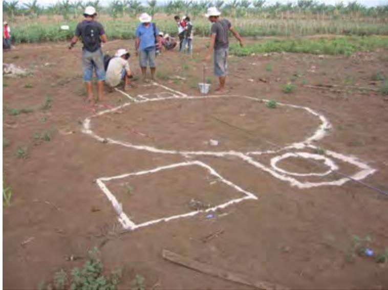
Gambar 191. Gambar lay out galian reaktor biogas
