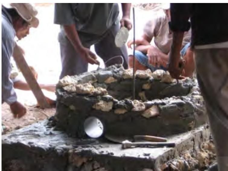
Gambar 137. Memasang dinding *inlet*
