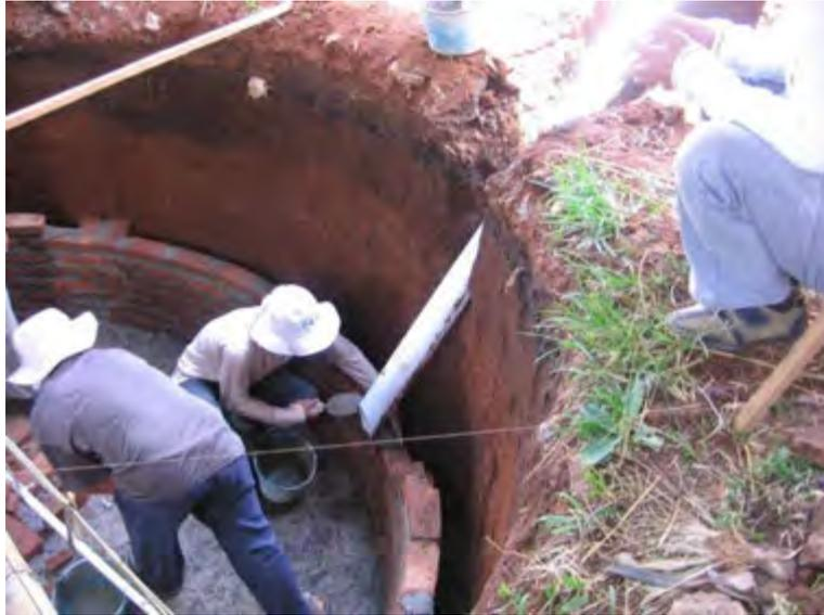
Gambar 65. Pemasangan pipainlet
