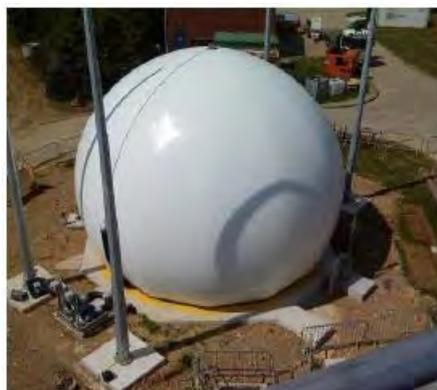
Gambar 14. Contoh reaktor biogas (Swedia)
