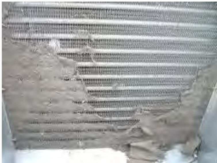
Gambar 3.2 Kondisi Koil Kondensor Sangat Kotor
